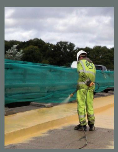
Britdex MDP is a 100% effective seamless bridge deck waterproofing membrane, flexible and robust enough to outlast the design life of many structures.
