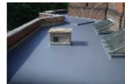
Uninsulated Roof Overlay
