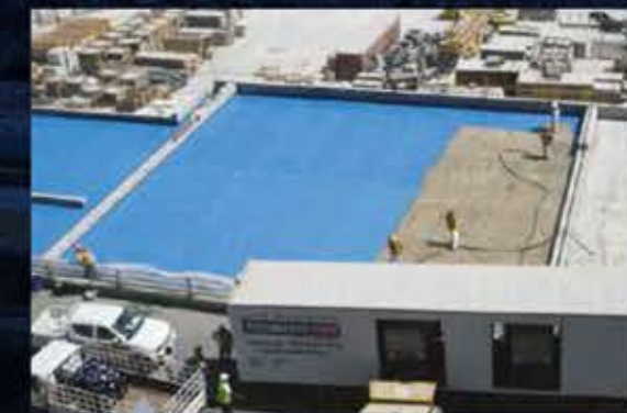
158,000m 2 of PmB Waterproofing applied to Al Sowah Island, Dubai UAE.
