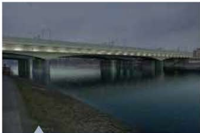
Project: Rontal Bridge, Lucerne, Switzerland Product: Kerb and drainage units Client: Basler & Hofmann
