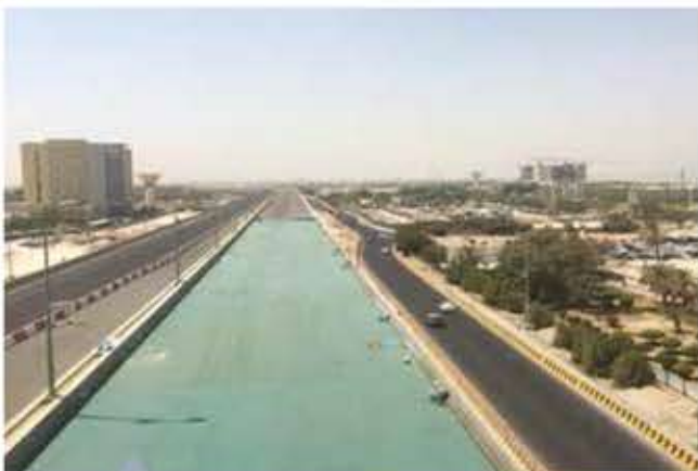
Project: RA167 Jamal Al Naser Street – Construction, Completion and Maintenance of Roads, Overpasses, Storm Water Drainage, Sewer and Other Services Client: Ministry of Public Work - Kuwait Main Contractor: ROBT JV
