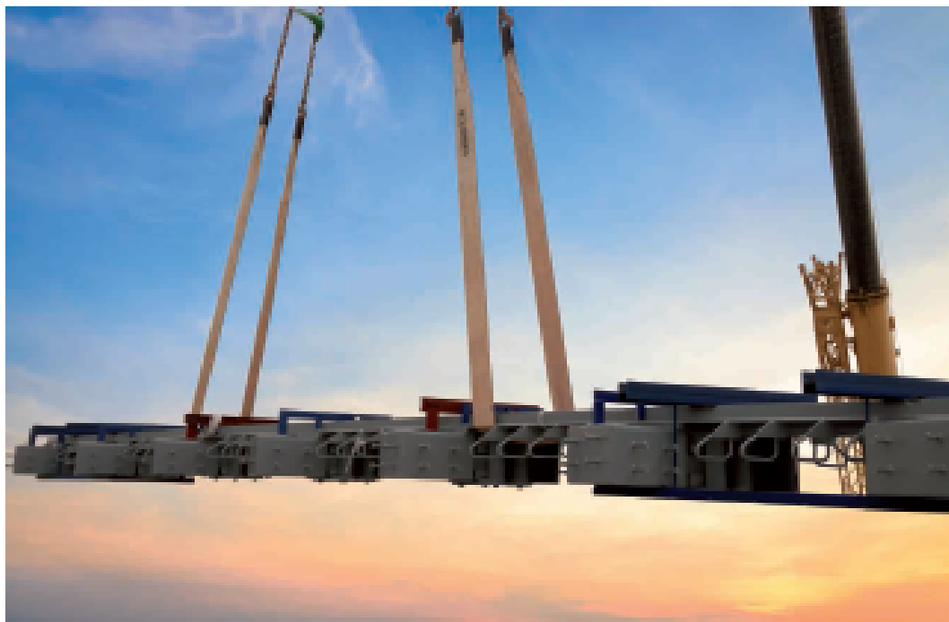
Installation of AR-EX Expansion Joints
