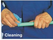
2. Before welding, pipes and fittings must be cleaned (to remove dust, grease, etc.) and dried.
