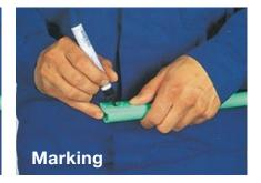
3. Mark the required depth of pipe insertion into the fitting (for a given outer pipe diameter - see the table).
