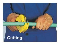
1. Pipes should be cut down to required length, at 90°C to the axis, using appropriate tools (pipe shears or cutters).
